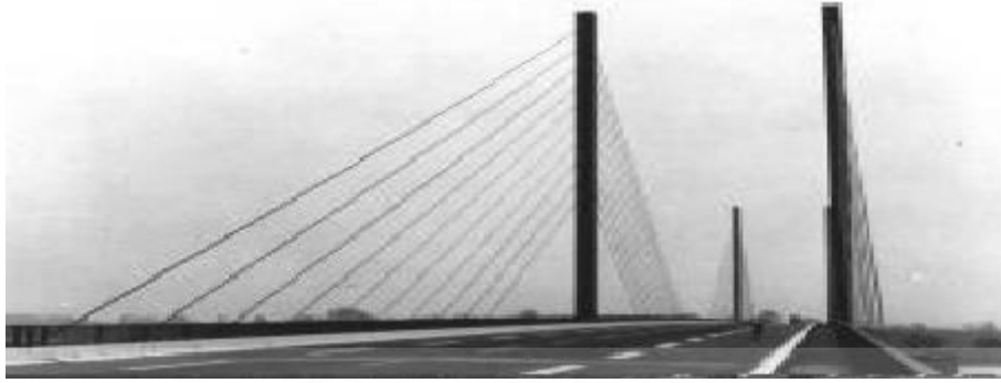
Fig 2.4 The Rees Bridge.
