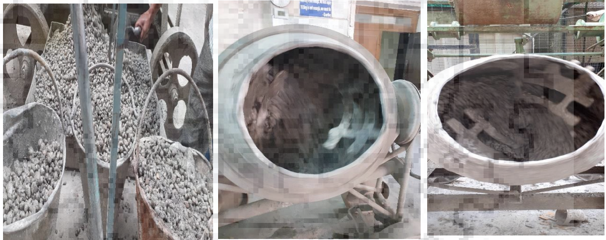
Plate 14 Mixing of concrete
