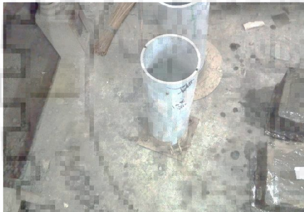
Pipe fixed upon the mould
