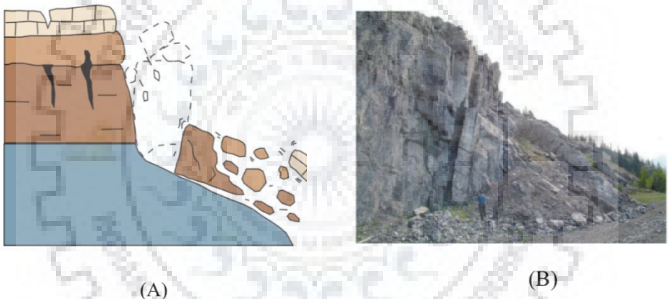
Figure-9 A rockfall/slide that occurred in Clear Creek Canyon, Colorado, USA, in 2005, (Photograph by Colorado Geological Survey.)
