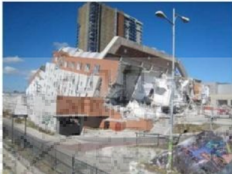
Figure 2.4 Overall view of collapsed building in Alto Rio [17]
