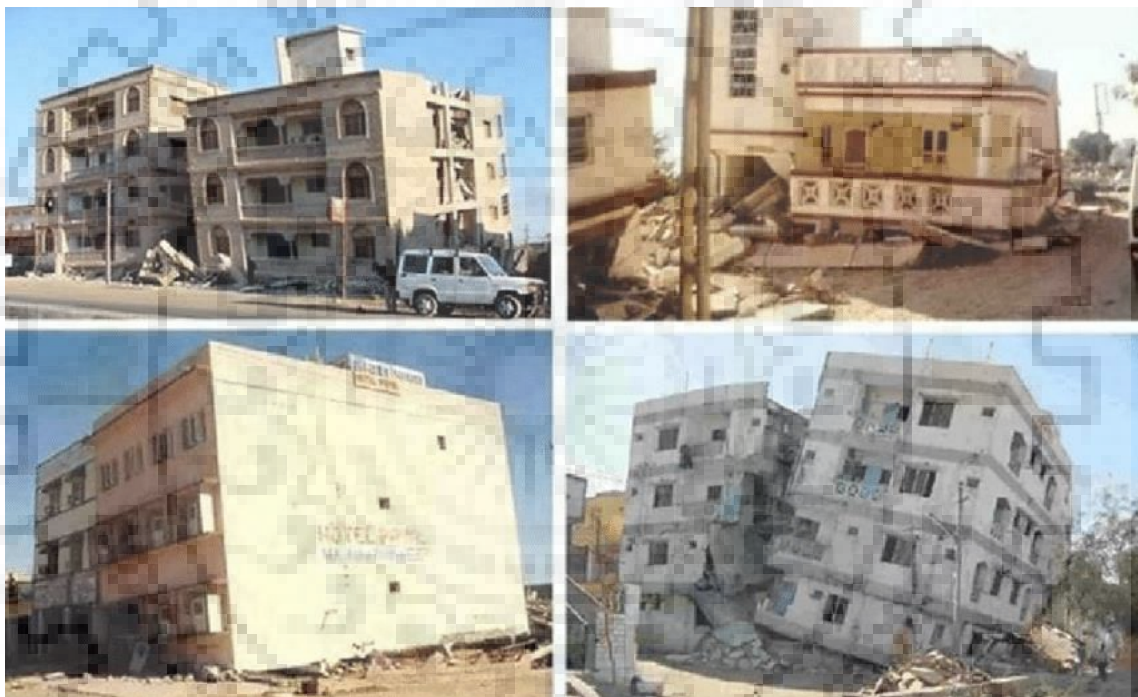
Figure 1.1 Failure of buildings with Soft Storey during Bhuj Earthquake, (2001).(IITK.ac.in)
