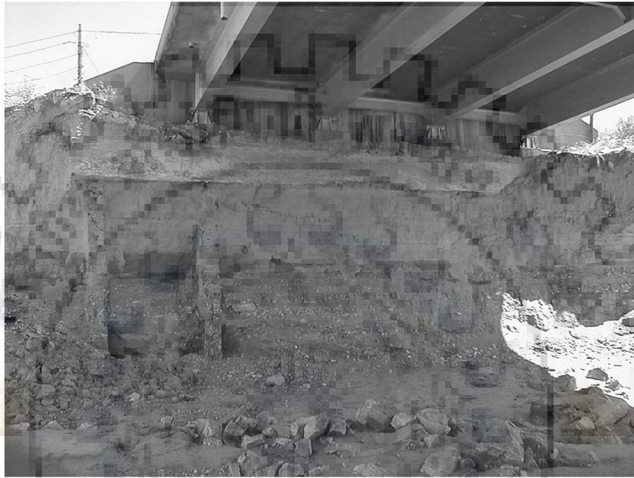
Figure 1.5 Field example of spill slope failure at a spill-through abutment at Cottonwood Creek, (Ettema et al. 2015).
