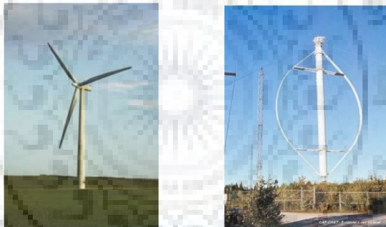
Fig. 2.1: Horizontal and Vertical axis wind turbine [14]
