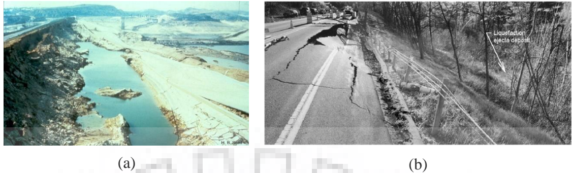
Fig. 1.1 (a) Lower Van Norman dam failure, California (Seed et al. 1973); (b) Road embankment failure during the Au Sable Forks earthquake in New York (Gingery 2003).
