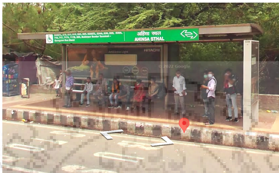
Figure 4.10: Ahinsa sthal bus stop shelter
