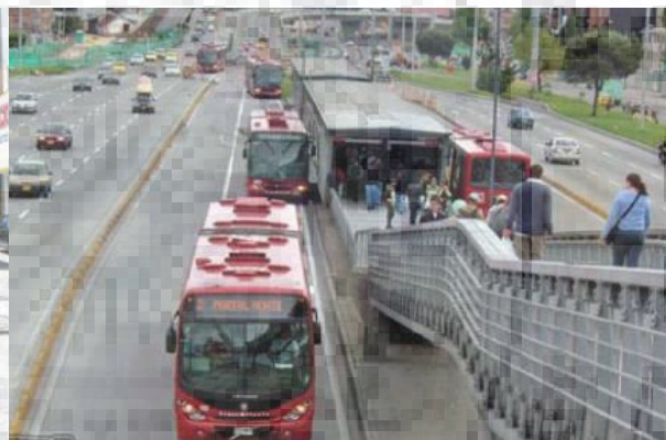
Figure 2.13: Bagota Transmilenio-Median Busways and Station
