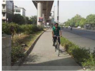
Figure 2.10: Bicycle lanes installed near Lajpat Nagar Metro Station, New Delhi
