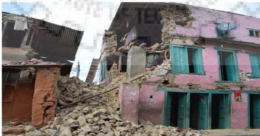
Fig 3.1 harm to the stone Brick work houses in Kangra (Source :- google.com)
