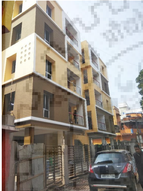
Figure 6.3 A multistorey building under construction in Khidirpur
