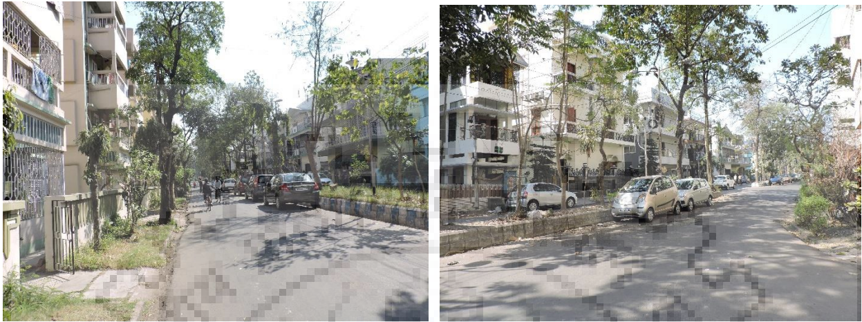
Figure 4.12 Residential area in Salt Lake Sector 1 (Source: author)
