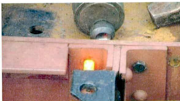
Figure 3.1- Hot-driven riveting process (Larsson, T. 2009)
