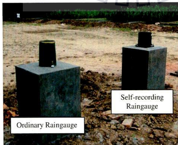
Fig. 3.8: Installation of Raingauges
