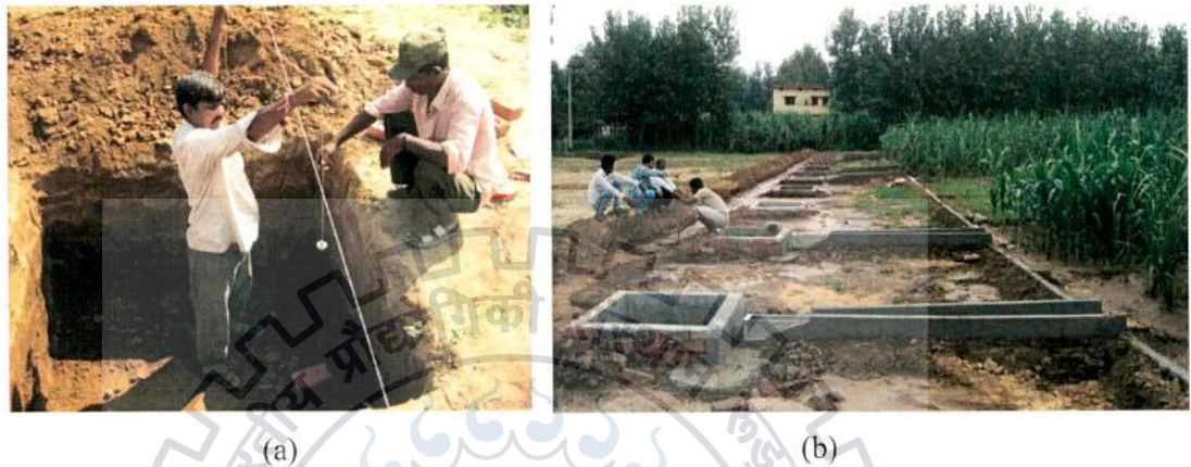
Fig. 4.4: Construction of collection chambers
