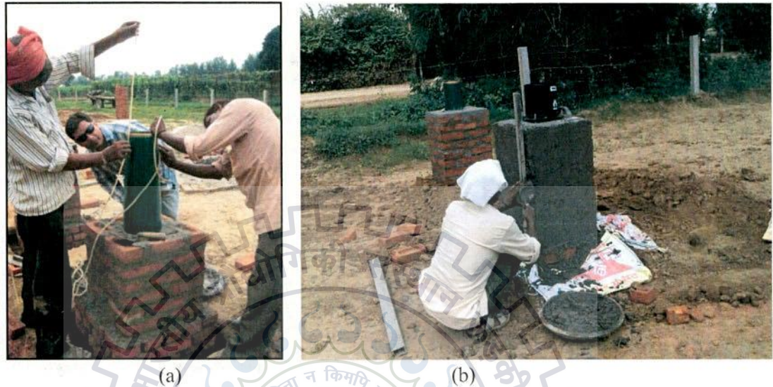
Fig. 4.6: Installation of Raingauges
