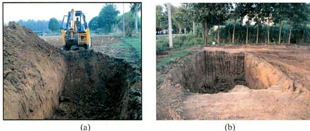
Fig. 4.3: Excavation of pond
