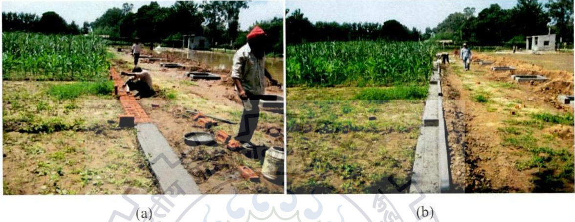
Fig. 4.9 Construction of plot boundary
