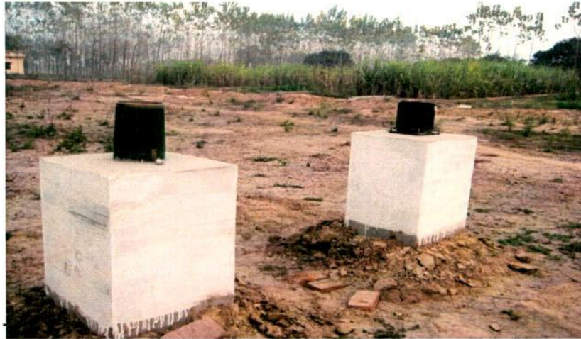
Fig. 4.13 Installation of ORG and SRRG
