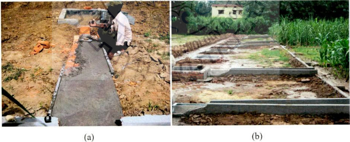
Fig. 4.10 Construction of approach channel
