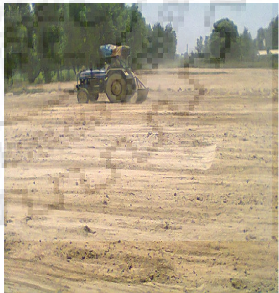
Figure 3.4 Addition of sandy soil to change the properties of parent soil
