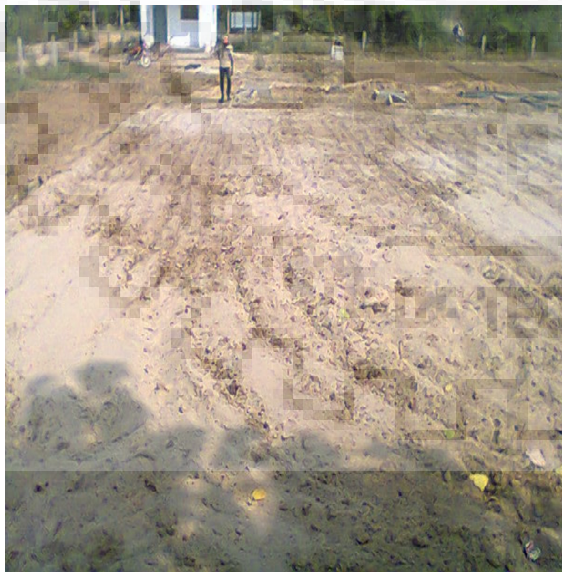
Figure 3.4 Addition of sandy soil to change the properties of parent soil
