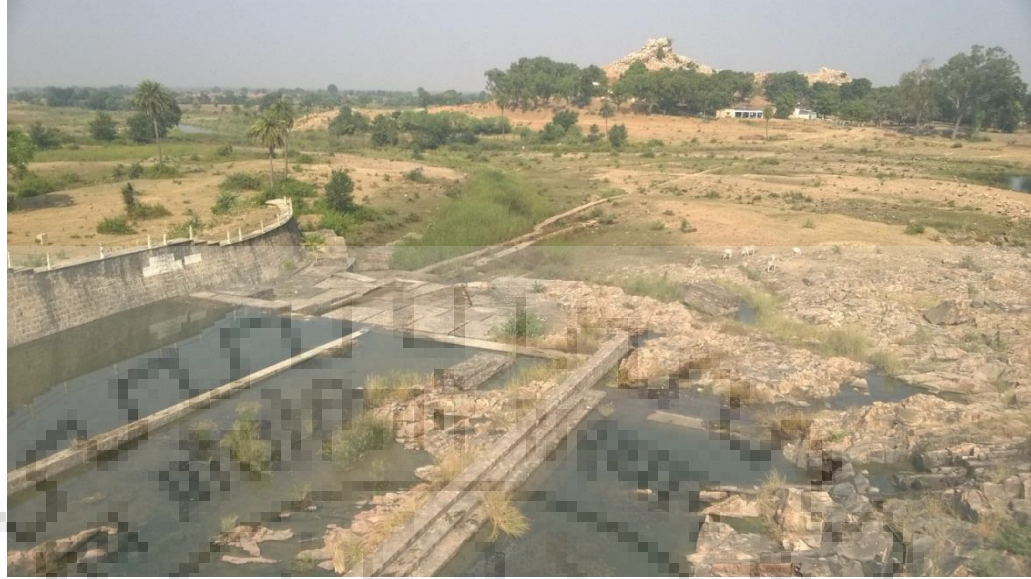
Place: Downstream view of Saprar Dam Latitude: 25.14°56'69.71"N Longitude: 79.8° 14. Elevation: 826 m
