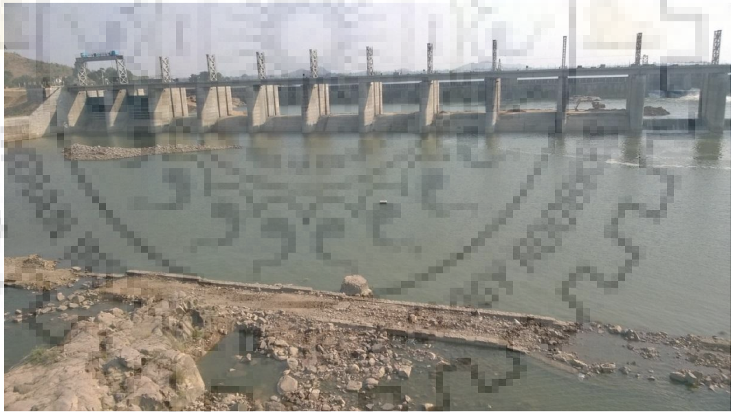
Place: Downstream view of Saprar Dam Latitude: 25.14°56'69.71"N Longitude: 79.8° 14. Elevation: 826 m
