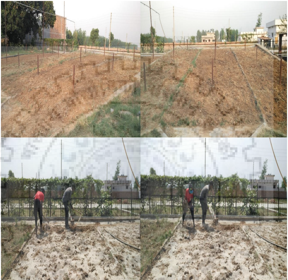
Addition of sandy soil by manual power.
