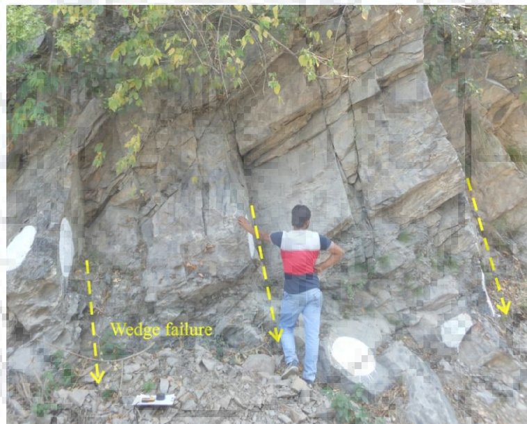
Figure 3.22: Blocky rock mass favoring wedge failure at slope S20
