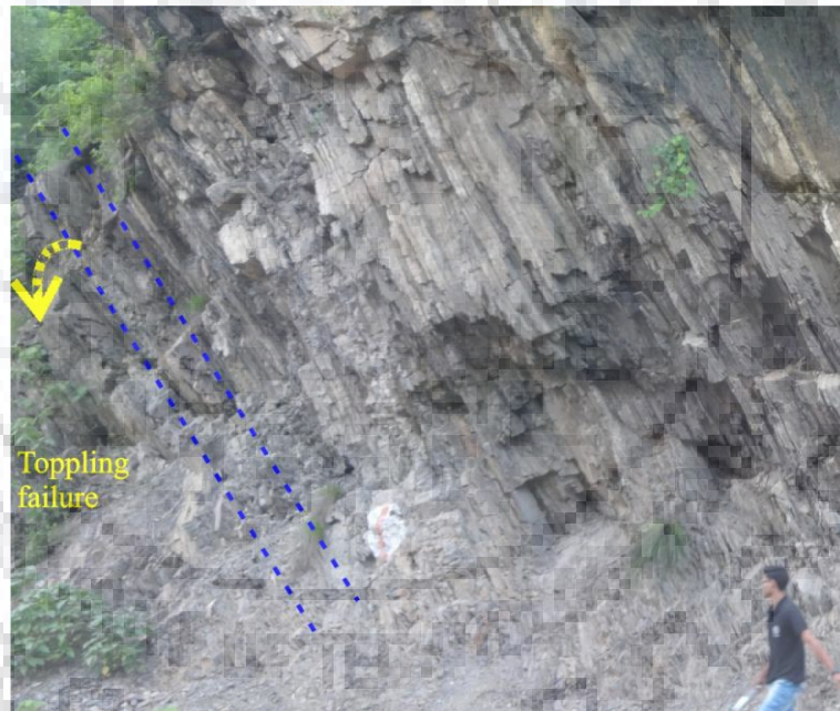
Figure 3.8: Steeply dipping discontinuities in Slate forming toppling failure at slope S6
