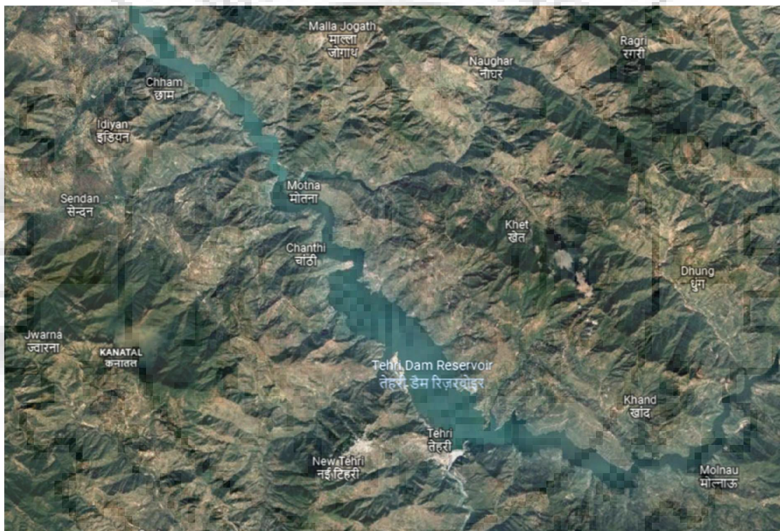
Figure 4.10: Tehri Reservoir (Source: https://www.google.com/intl/en_in/earth )
