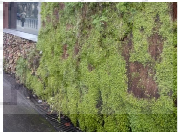
Figure 13 - Image showing green facade
