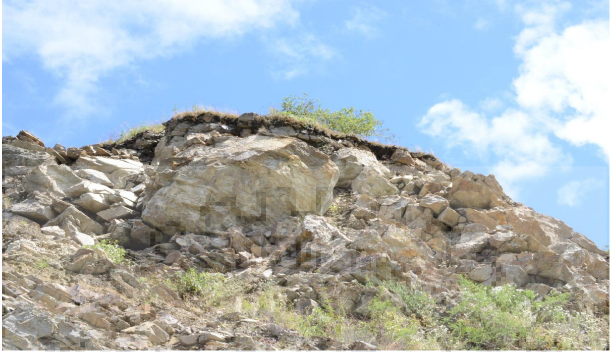
Figure 3.4: Detachment of rocks on site at the top of the landslide
