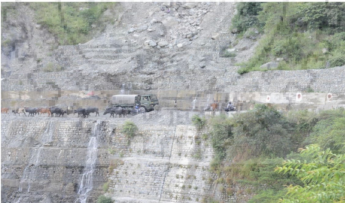
Figure 1.4: Drainage above the road in 2017 (Photo taken on 25 th September, 2017)
