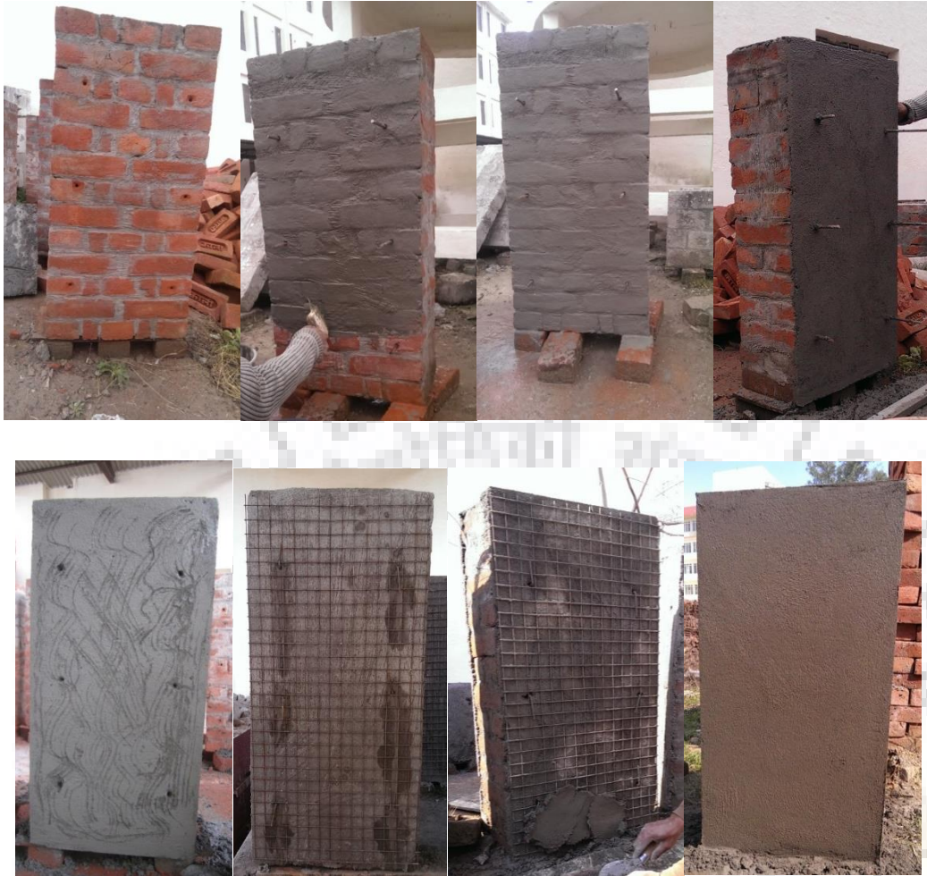
Figure 3. 1 : Stages strengthening unreinforced specimen with WWM
