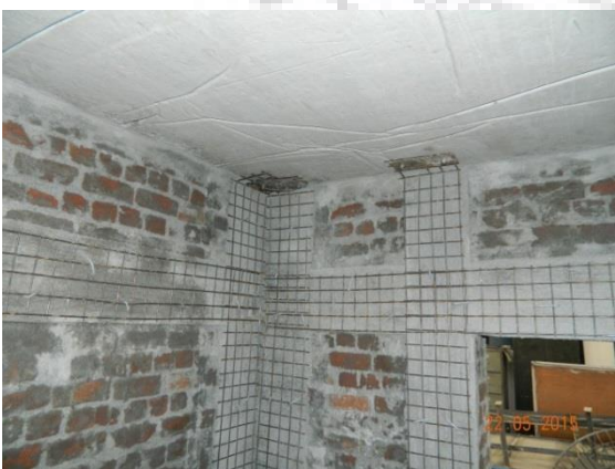
Figure 4. 12 : Model strengthening process
