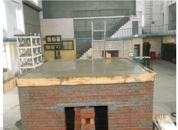
Figure 4.7 : Casting of roof slab
