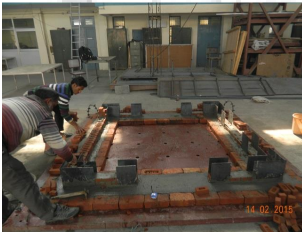
Figure 4.5 : Laying of bricks above foundation
