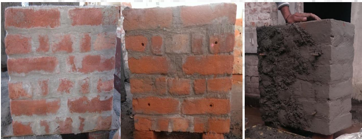
Figure 2. 3 : (a)-(b) Stages of strengthening unreinforced specimen with WWM (contd.)
