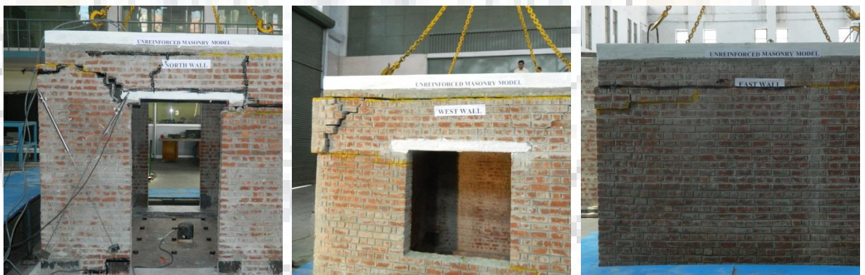
Figure 4. 22 : Failure pattern after second shake
