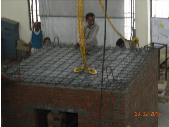
Figure 4.7 : Casting of roof slab
