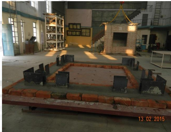
Figure 4.4 : Casting of foundation
