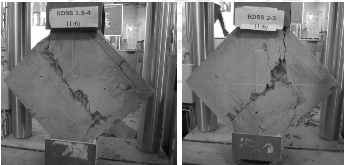
Figure 2. 7 : Low strength mortar (1:6) retrofitted panel with 1 inch, 1.5 inch and 2 inch spacing WWM
