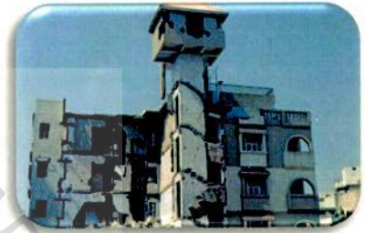
B) Traditional Bhunga that survived in Ludia village (≈70 km N of epicentre) Modern construction that collapsed in Ahemdabad (250 km E of epicentre)
