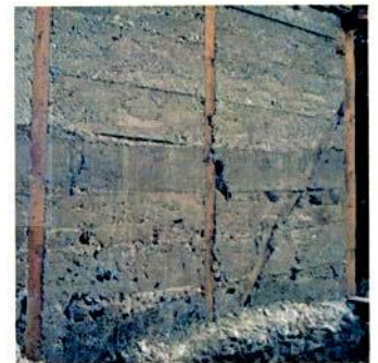
Fig.3.30. Various bracing patterns and masonry laid in concrete (Source: World Housing Report #146)
