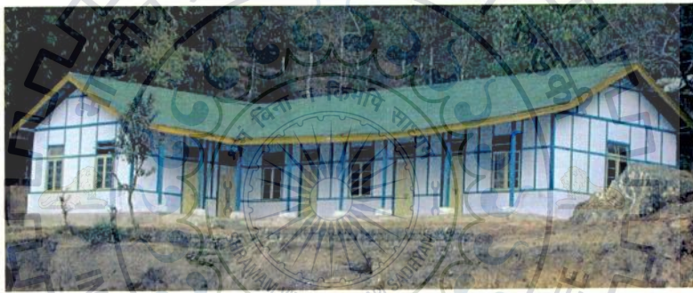
Fig.3.9. A school building in Assam made in Assam/Ikara style (Source: World Housing Report #154)
