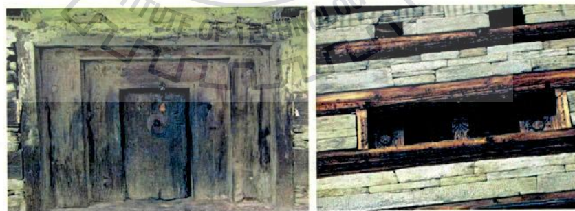
Fig.3.18. Small openings (Source: World Housing Report #150)
