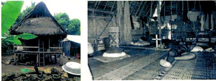
Fig.3.21. A) A Nicobarese hut on timber stilts and ladder for access (Source: Rawal.V, et.al) B) Interior of the hut showing perforated mat (Source: Sinvhal A., et al)
