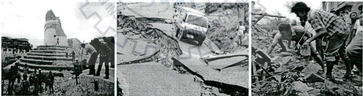
Figure 12: Damage during 2015 Nepal Earthquake in Nepal
