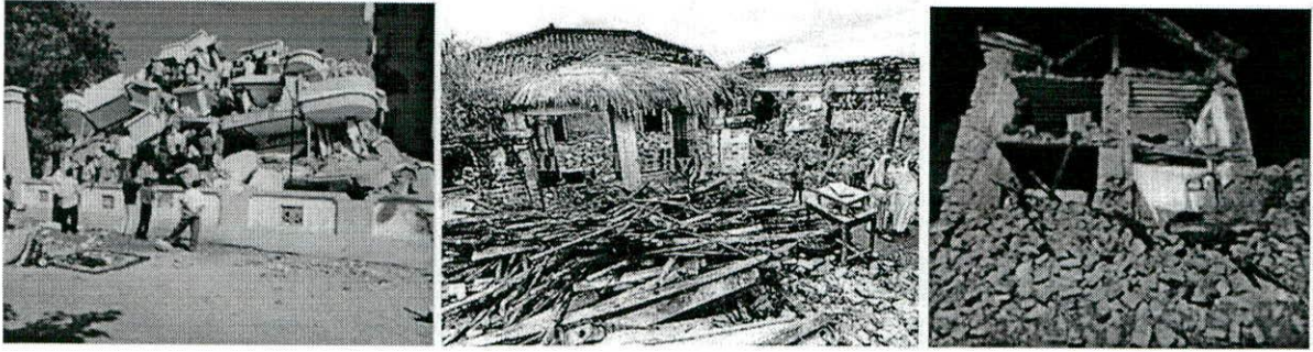
Figure 10: Damages during 1988 Bihar-Nepal Earthquake
