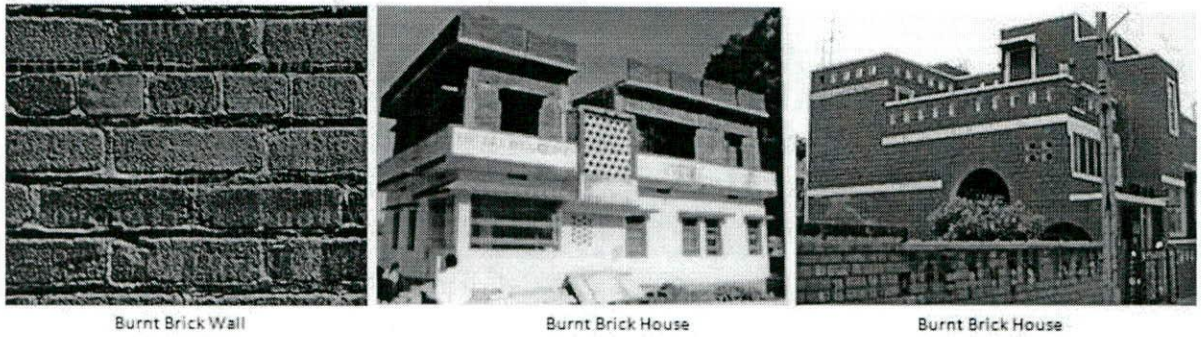
Figure 19: Type B House, Burnt Brick Wall
