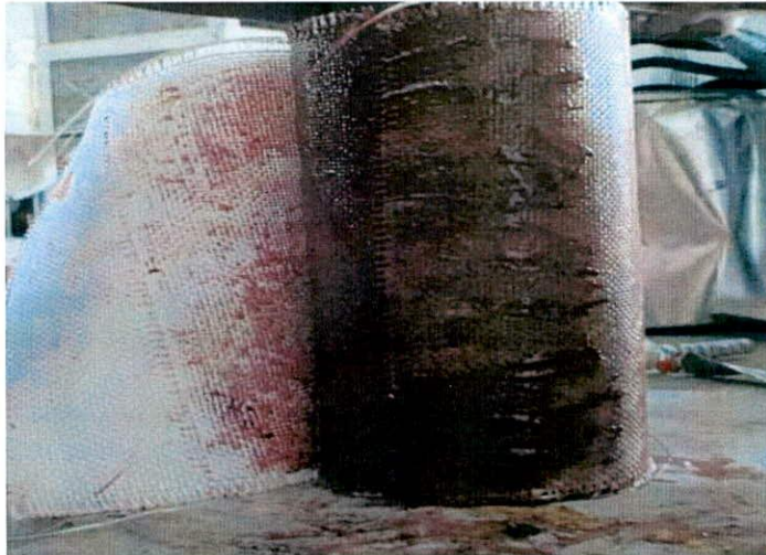
Fig 6.3: wrapping of FRP and saturating with epoxy resin
