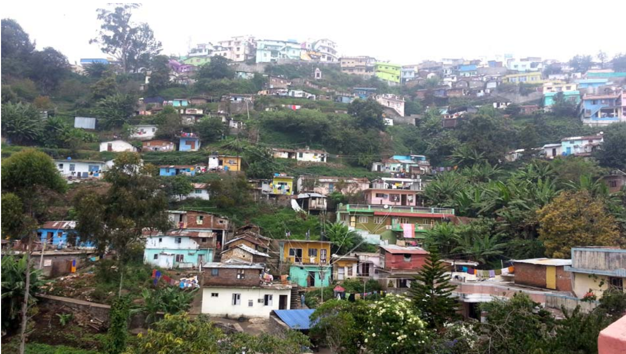
Fig 5.16 Urbanization on the steep slope of the Gandhipuram Slope, Facet no. 34
