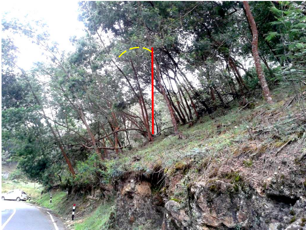
Fig 2.18 Tilted Trees along the Pillar Rocks Road
