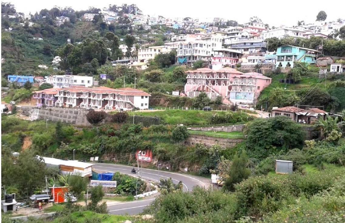
Fig 5.13 Ananthagiri Slope 1 showing heavy urbanization on the slope
