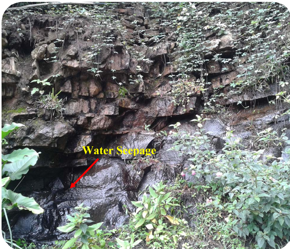
Fig 5.26 Water dampening the highly jointed rock exposure in Pudukkad Slope
