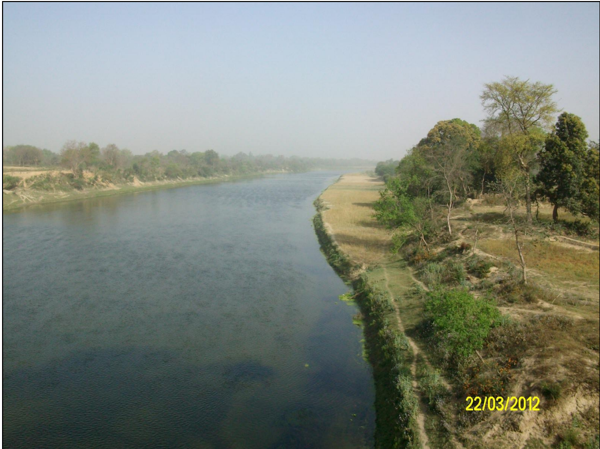
Figure 2.2 Upstream view of the active channel of the Gomati River at Haidergarh.
