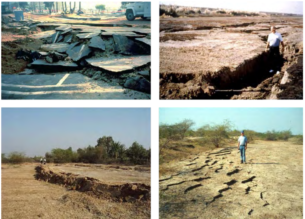
Figure 1.5: Terrain deformations due to the Bhuj 2001 earthquake (ISR 2007).
