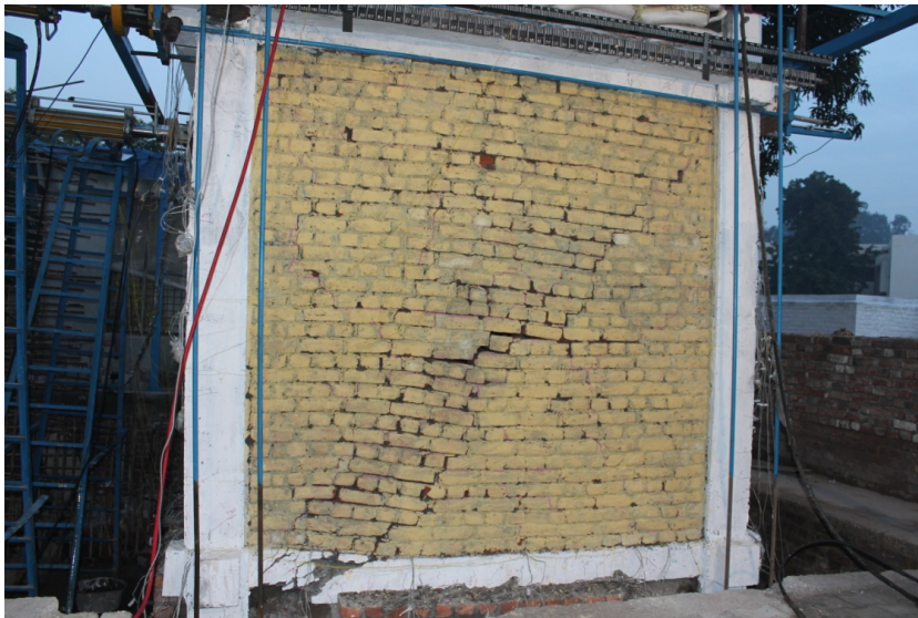
Fig. 3.3 View of the In-plane wall after the test
