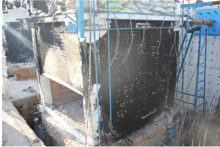
Fig.3.26: A view of the frame after residual test
