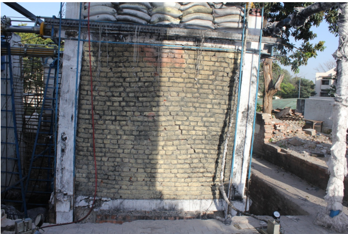
Fig. 3.25: The test frame during the residual load test.
