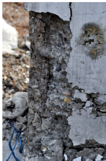
Fig. 2.65: (a) Damaged core concrete in Beam B7 (b) failed shear stirrup in beam B7 (c) view of a column
