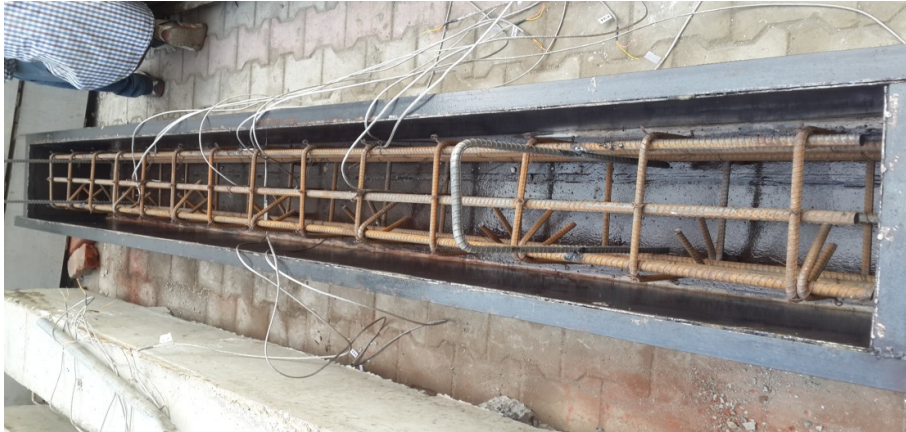
Fig. 4.2: Reinforcement cage with thermocouples in mould.
