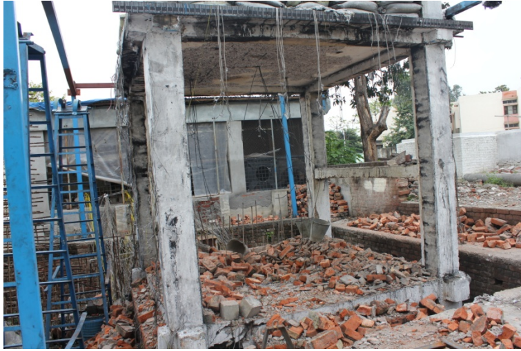
Fig. 3.29: A view of the frame after removal of infill walls
