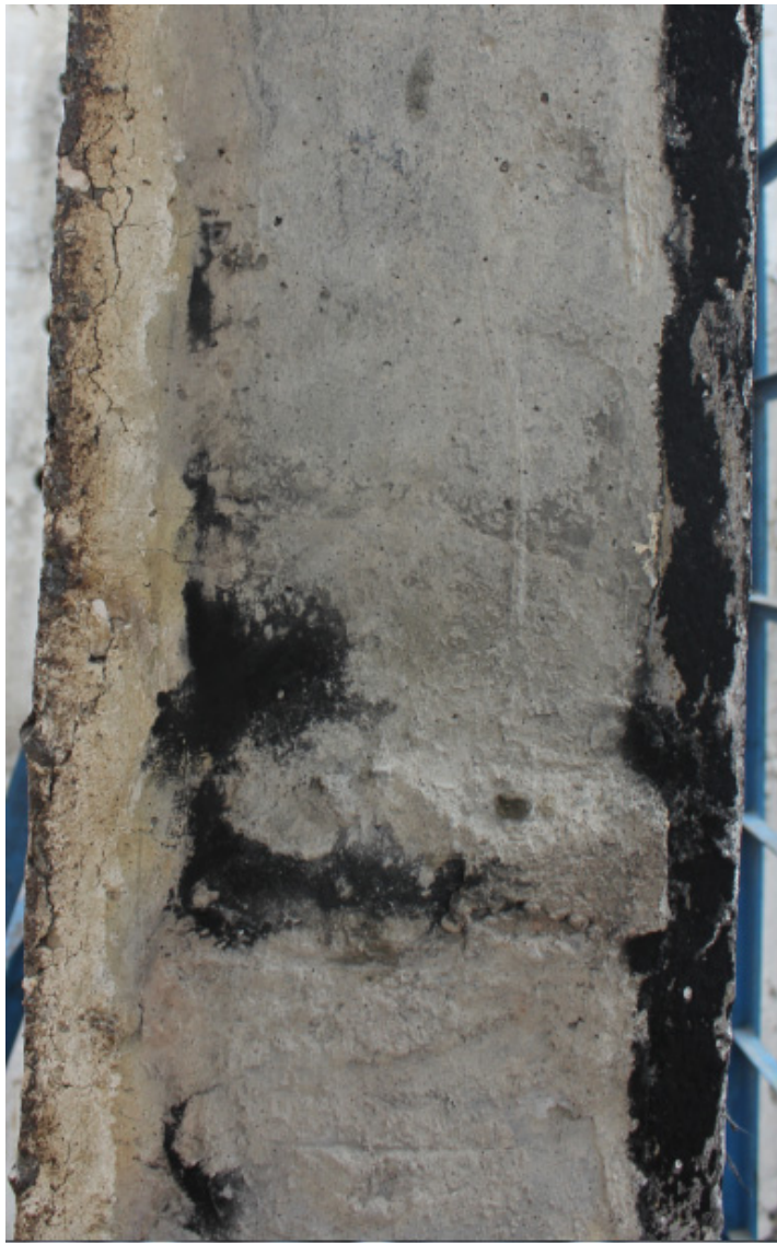
Fig. 3.30: Column C4 after removal of infill walls
