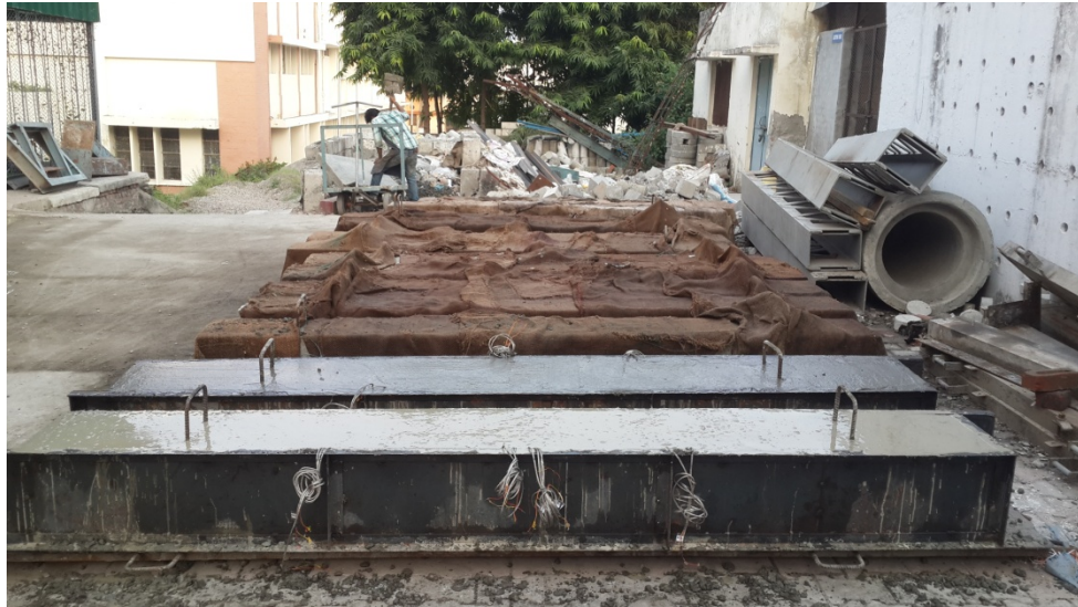
Fig.4.4: RC columns after casting.
