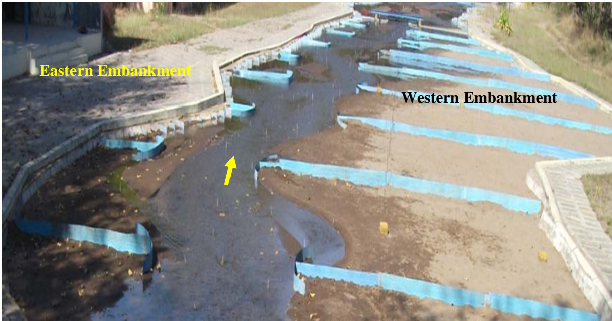
Figure 7.24 b) Closer view - Flow touching the wings of T-shape groynes, but no shoal flushed or sediment motion.
