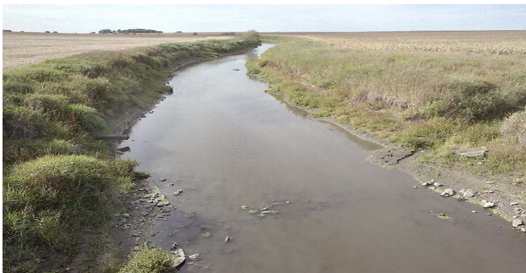
Figure 2.14 A channelized section of the South Fork of the Crow River in Meeker County, Minnesota (Wikipedia)
