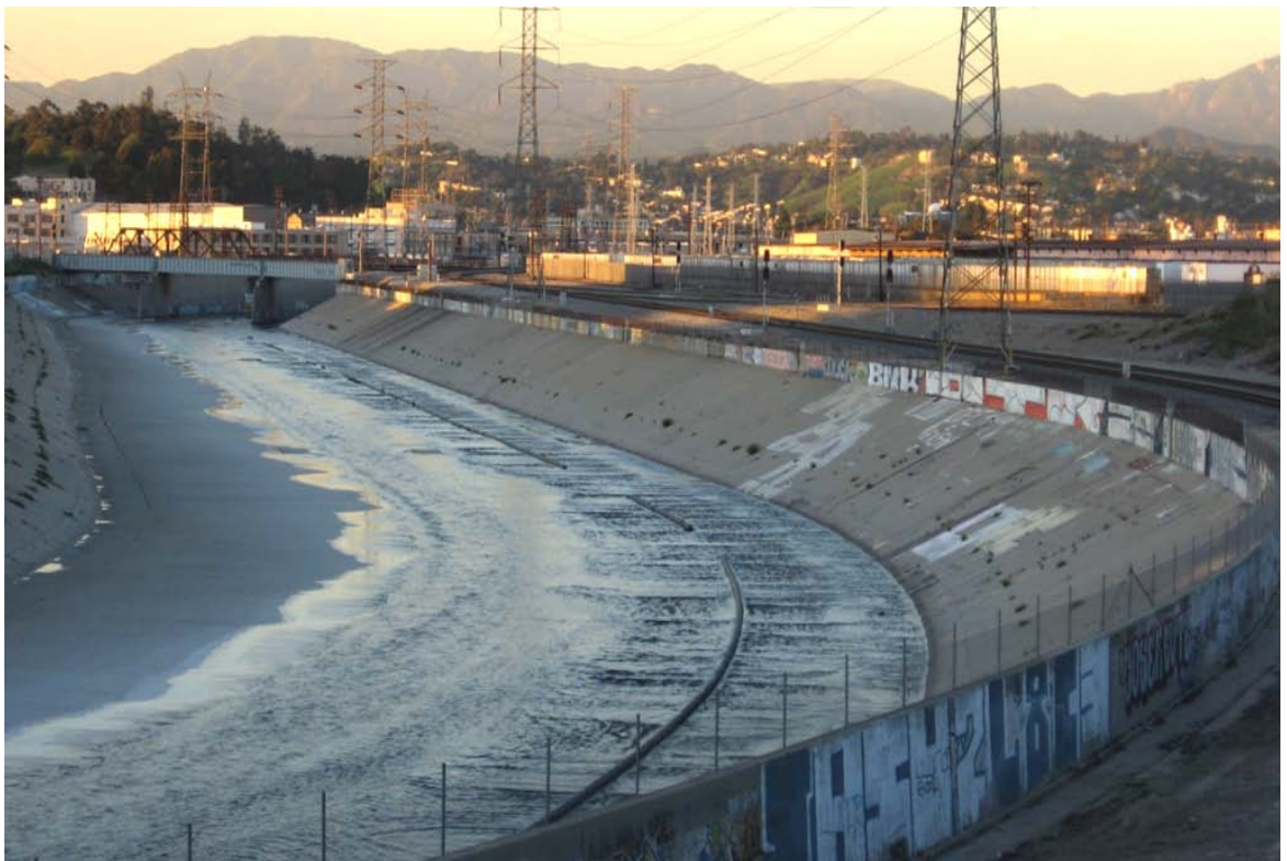
Figure 2.12 The Los Angeles River is extensively channelized with concrete embankments (Haltiner et al., 1996)
