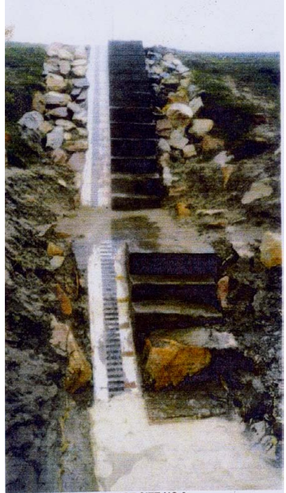
Figure 7.3 Gauge site at Bhaptiahi
