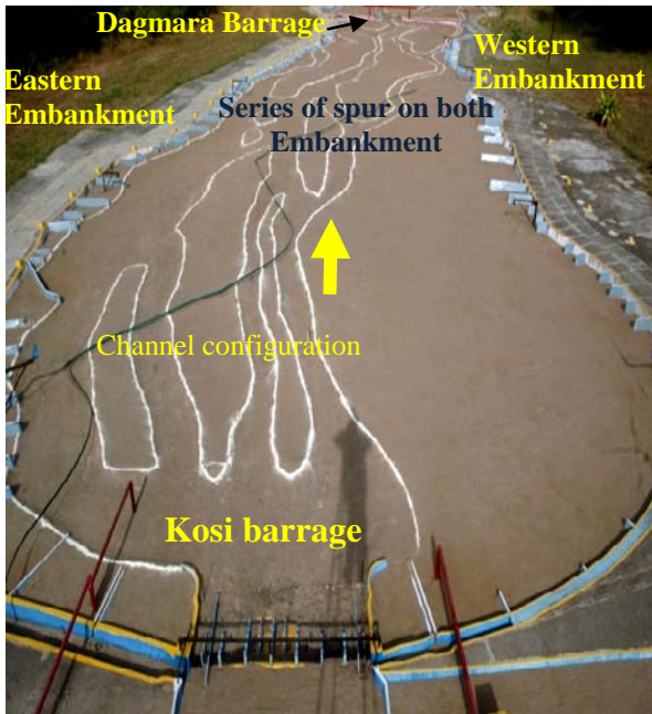
Figure 7.11 View from upstream end and from Kosi barrage to Nirmali
