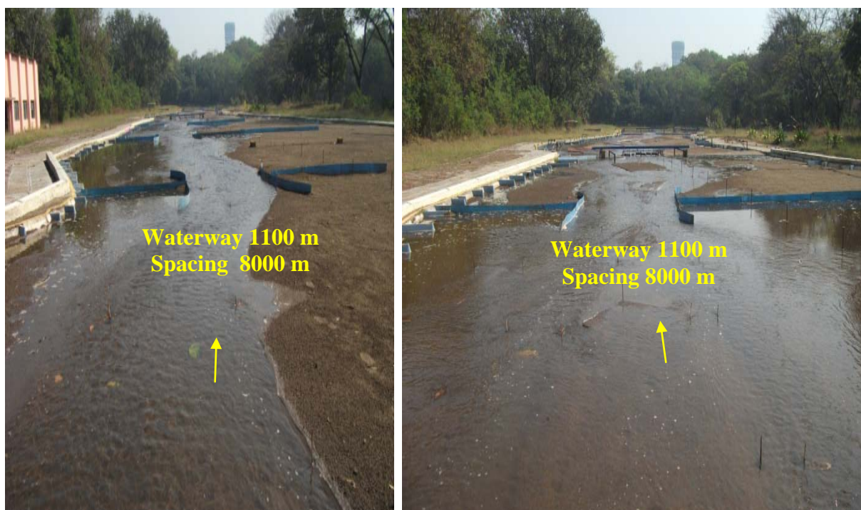
Figure 7.31 Closer view showing water is flowing haphazardly
