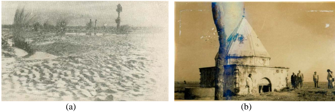
Figure 3.6 Effect of flood a) Enormous silt-the aftermath of flood (1954) b) Temple silted up to its arch. (CWPRS record)
