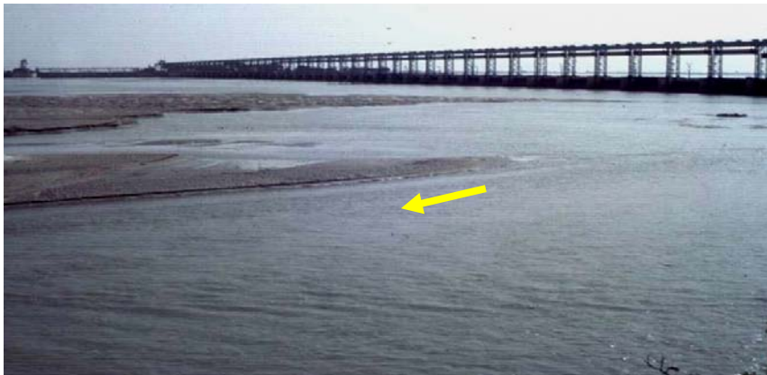
Figure 3.10 Kosi Barrage (downstream view)
