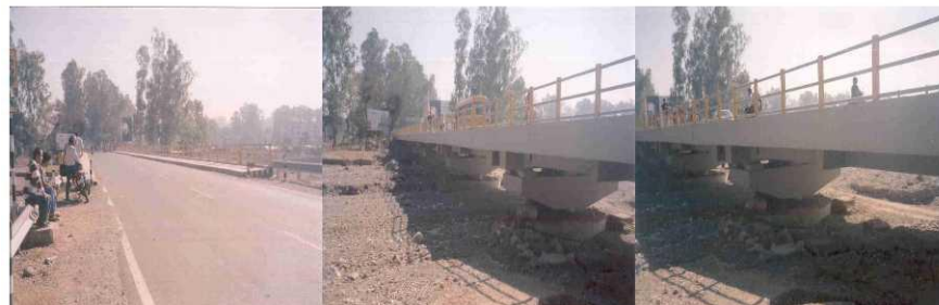
Fig 6.51: Photographs of Bridges of 7.5 m Road Width and Steel Railing
