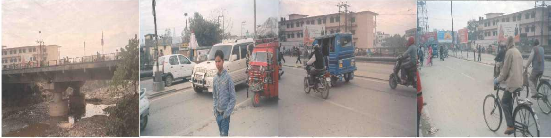
Fig 6.56: Photos of Bridge of More than 10 m Length and with Divider
