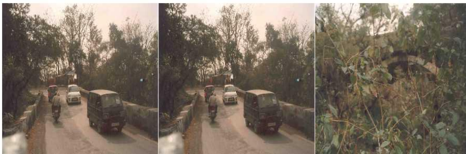
Fig6.45: Photos of a bridge on River Tons
