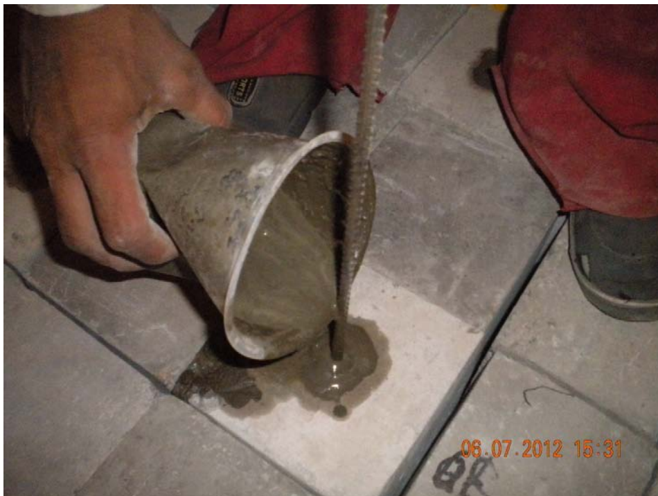
Fig. 3.9 Grouting of bolts
