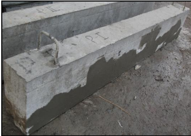
Fig. 3.12: A honeycombed beam specimen after repairs
