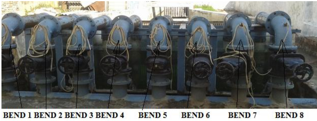
Figure 3.13 Bend meters, valves and manifold of the model
