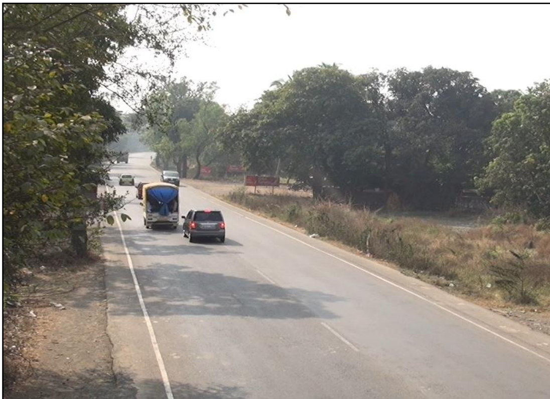
Figure 6.5 Sample image of section T-12 with paved shoulder
