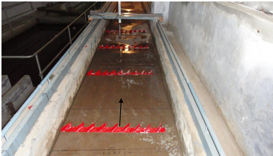
Fig. 4.9 Four arrays of installed vanes
