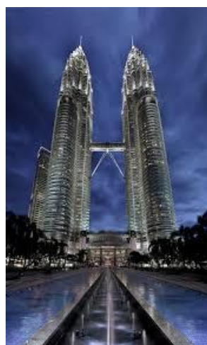
(h) Petronas Tower
