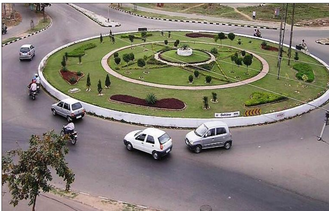
Figure 1.5 Roundabout in Chandigarh city, India (March, 2013)
