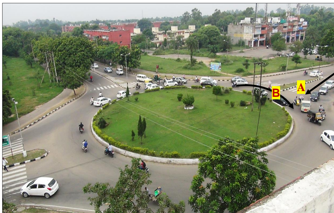
Figure 3.5 Markings at entry and circulating section of a roundabout for flow measurement
