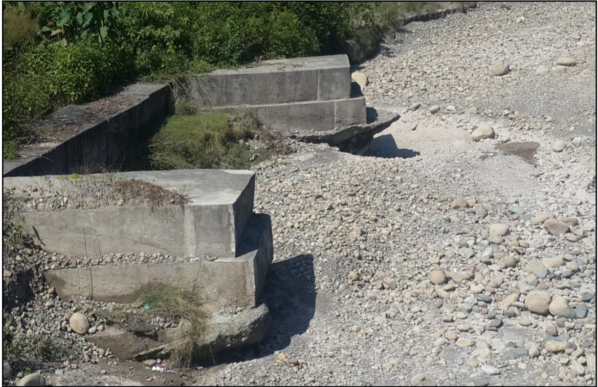
Fig. 1.3 Spur dikes installed at river Bhakhra near Haldwani, Uttarakhand (India)
