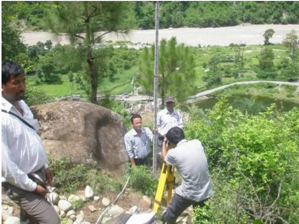
Figure 3.4 Transferring the datum from a kilometre stone to the RBF site
