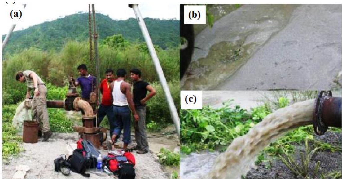
Figure 3.6 Well development process: (a) Pumping at high rate (b) sand abstracted out from the well (c) water mixed sand from the production well
