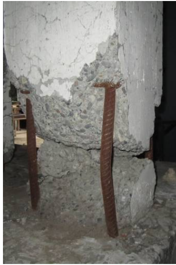
(b) Buckled reinforcement
