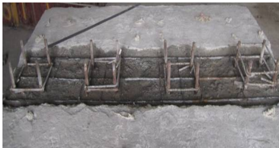
(a) Foundation after removing the columns
