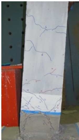
(a) Flexural cracks in beam
