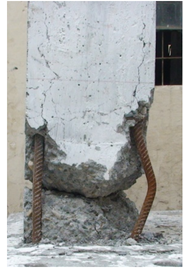
(b) Buckled reinforcement
