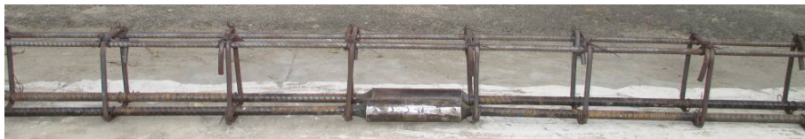
(a) Rebar connection using coupler at center in CB 102 and CB 122
