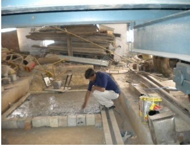
Photograph 4.12 Finished Surface of HSHPC Pavements
