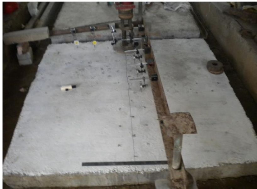
Photograph 4.22: Failure of 160 mm Thick HSHPC Pavement at Edge during Testing
