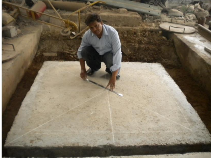
Photograph 4.15 Preparation for Pasting the Studs
