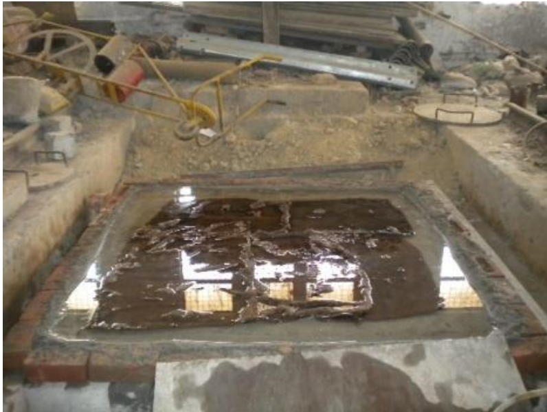
Photograph 4.13 Curing of HSHPC Pavement
