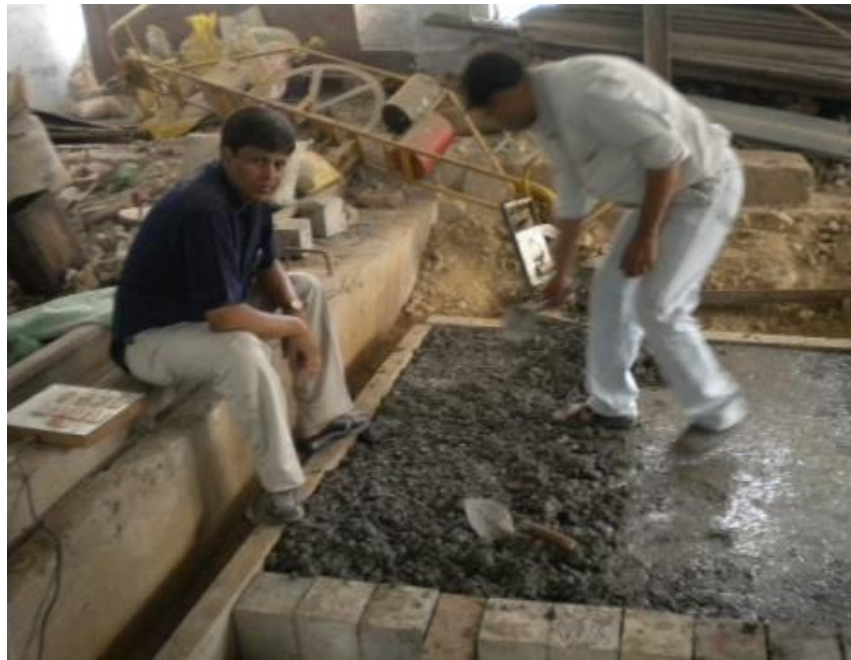
Photograph 4.11 Laying of HSHPC Mix for Pavements
