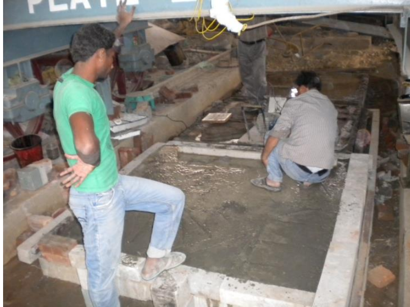
Photograph 4.14 Three HSHPC Pavements Cast for Investigations
