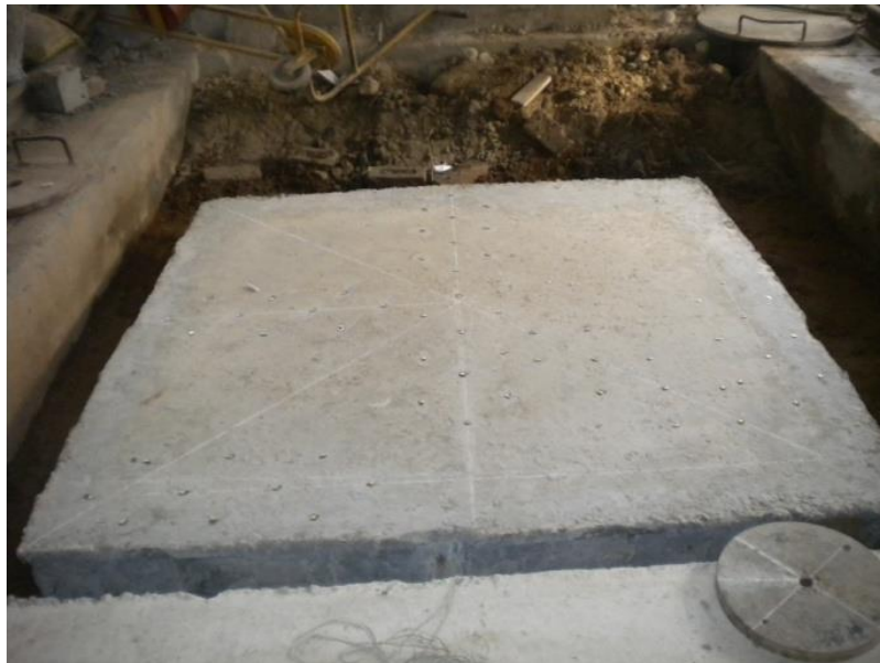
Photograph 4.16 Studs on Surface of HSHPC Pavements
