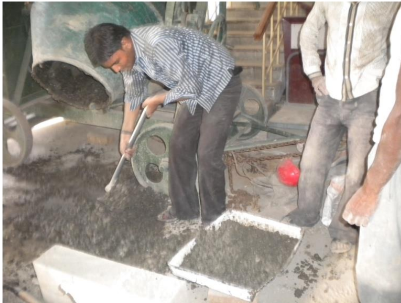
Photograph 4.1 Mixing Process of HSHPC Mix
