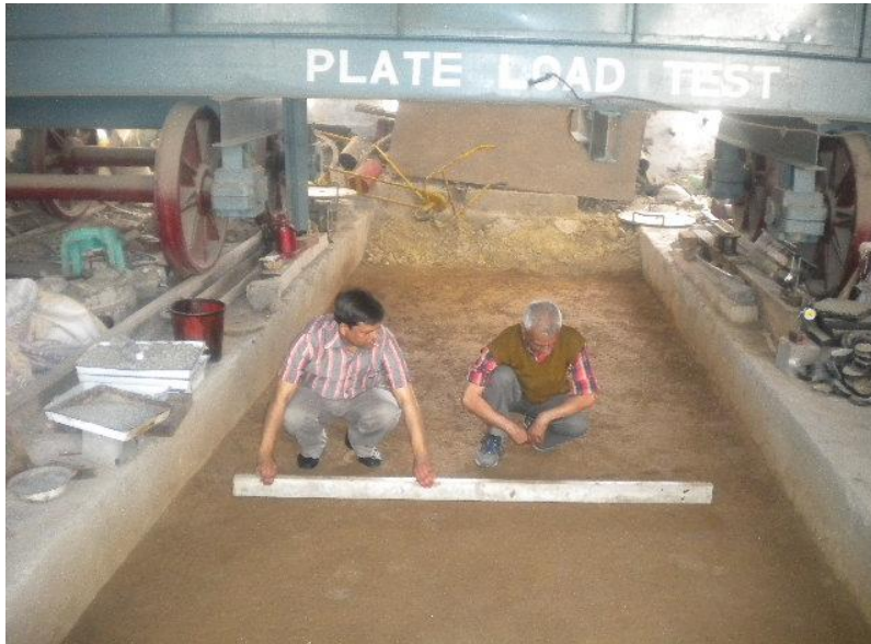
Photograph 4.10 Preparation of Soil Subgrade for Laying of HSHPC Pavements
