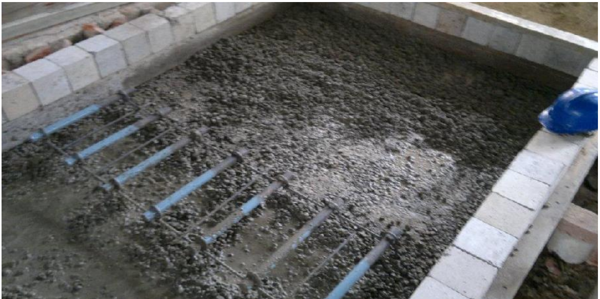
Plate 3.26 Laying of PQC
