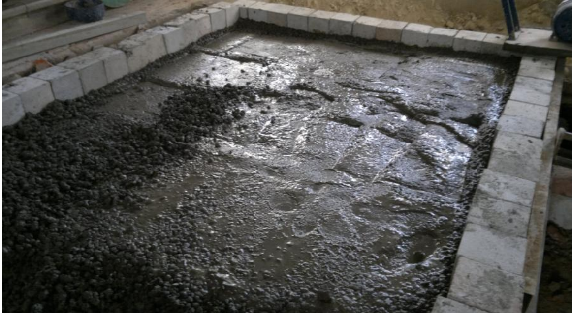
Plate 3.27 Layer Wise Compaction Performed on Fresh PQC
