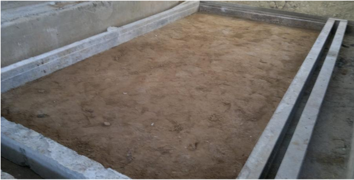
Plate 3.23 Compacted subgrade and installed form work
