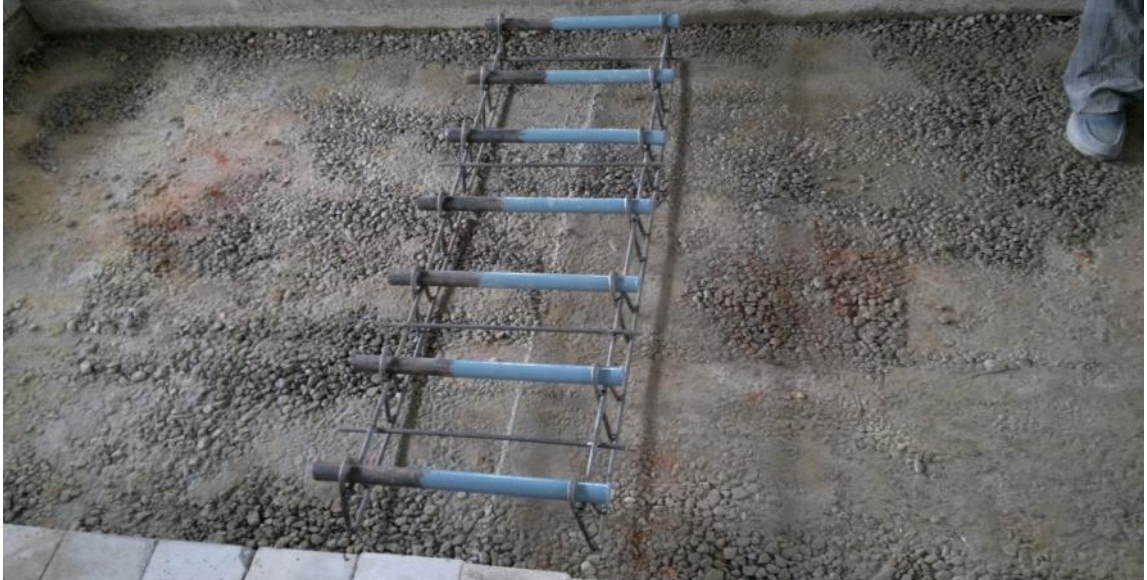
Plate 3.25 Positioning of Dowel Bars
