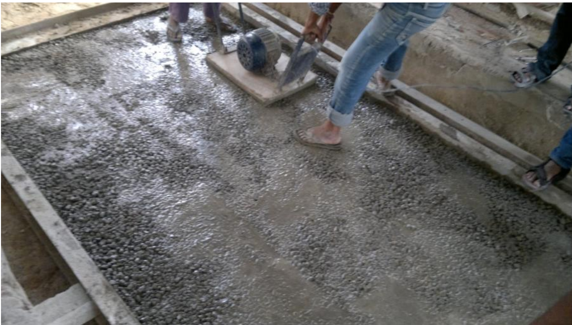
Plate 3.24 Finished DLC surface
