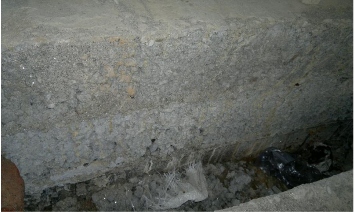
Plate 3.29 Finished Thickness of Rigid Pavement Prototype
