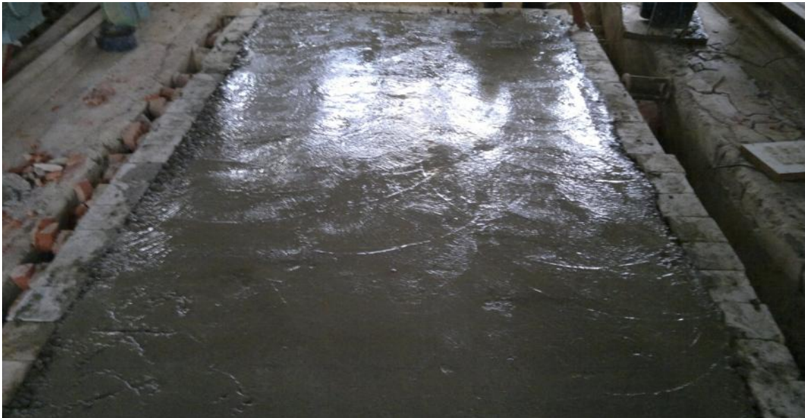
Plate 3.28 Levelled PQC Surface
