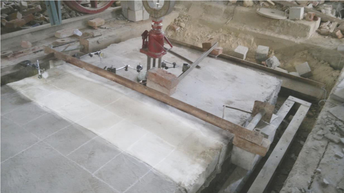
Plate 5.3 Plate load test on WMF reinforced rehabilitate PQC
