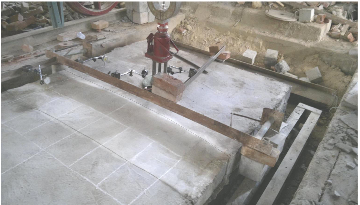
Plate 5.2 Plate load test on normal concrete rehabilitated PQC
