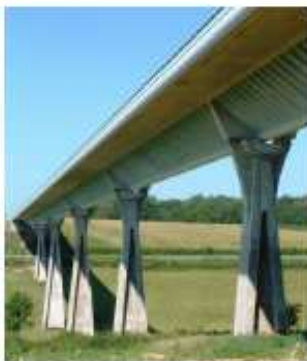
Maupre Valley Viaduct, Charolles, France
