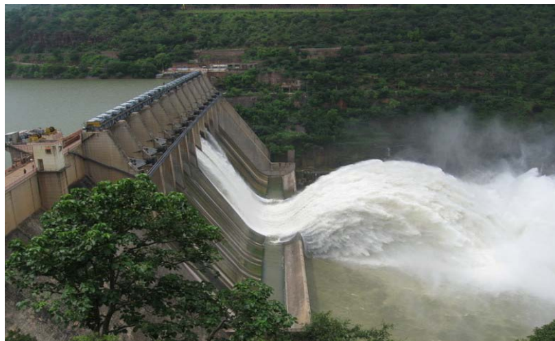
Fig. 1.3 Water release through hydraulic structure of the Krishna River in Srisailem Dam, Andhra Pradesh, India
