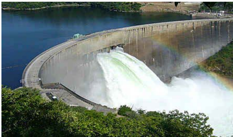
Fig. 1.4 Water release through hydraulic structure of the Zambezi River in Kariba Dam, Zimbabwe
