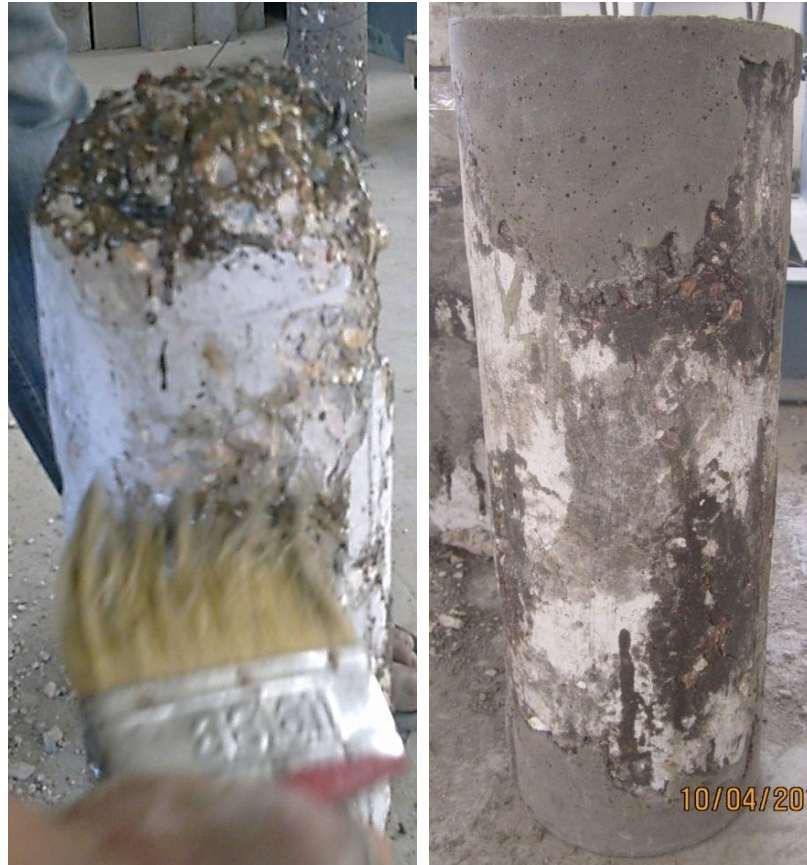
Fig. 2. 10: Application of bonding agent and application of micro concrete
