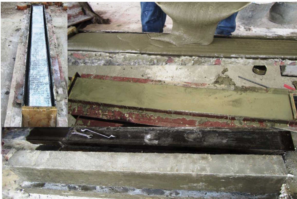
Fig. 4.9: HSFRC jacketing in progress
