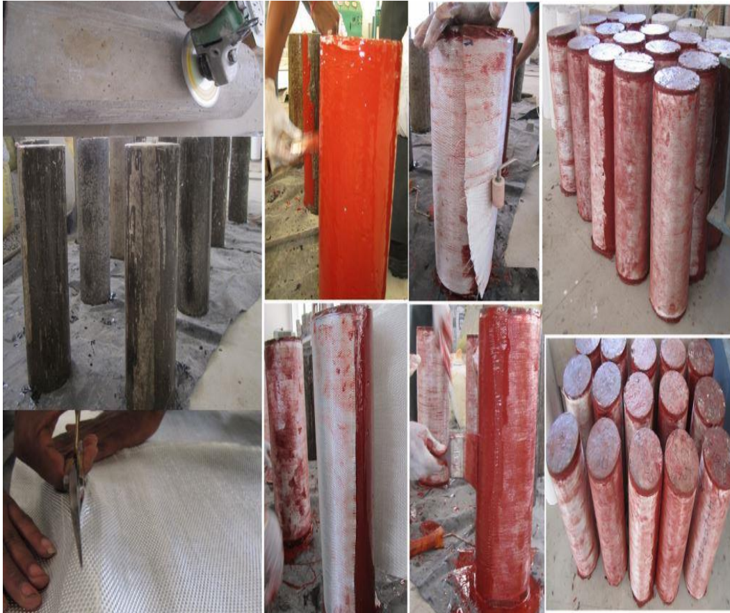
Fig. 2.13: Stages of GFRP jacketing
