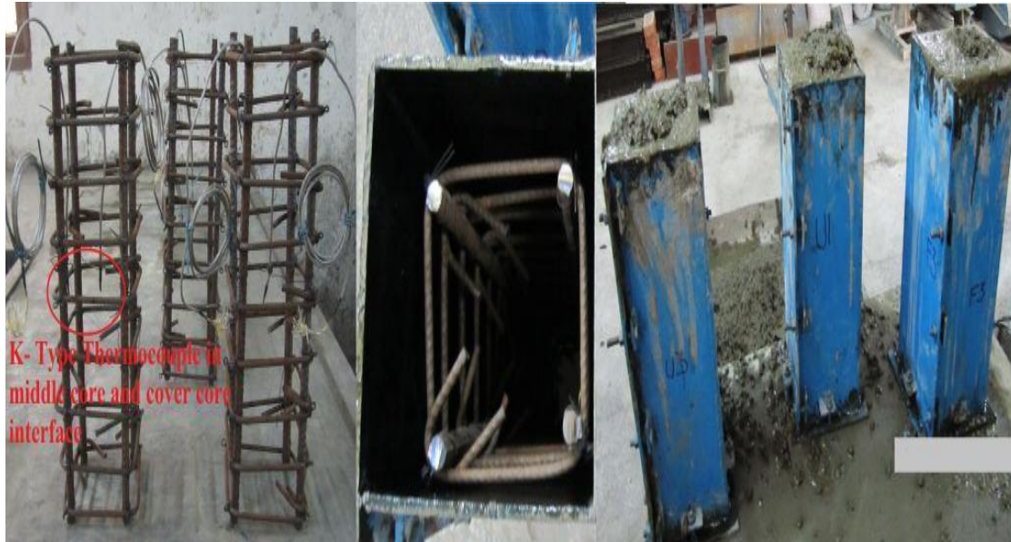
Fig. 3.3: Stages of thermocouple binding, reinforced gauges placed inside formwork and casting of square specimens
