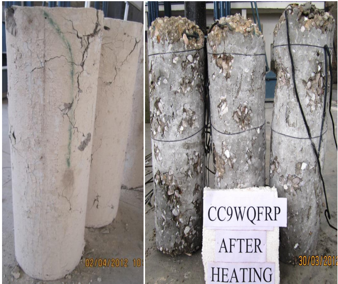
Fig. 2. 8: Surface cracking and spalling observed in test specimens exposed to 900 °C and cooled naturally and water quenched
