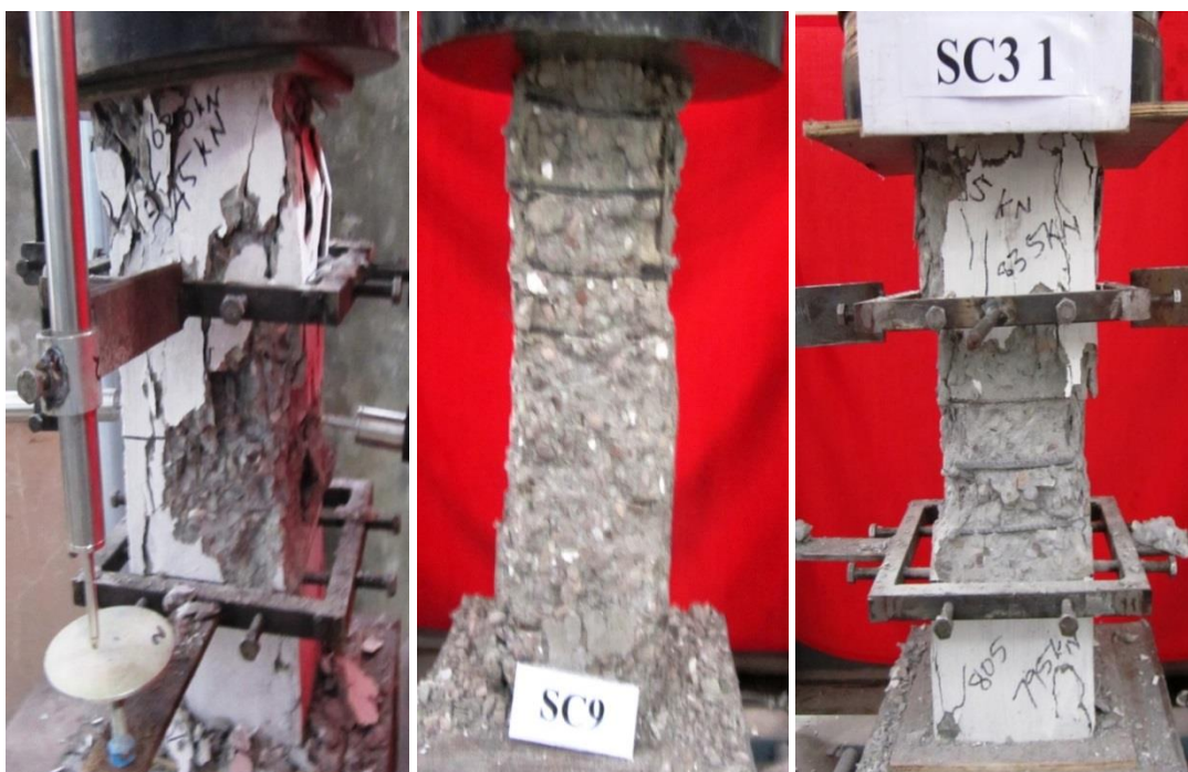
Fig. 3.12: Typical crushing failure of control and heat damaged square short columns
