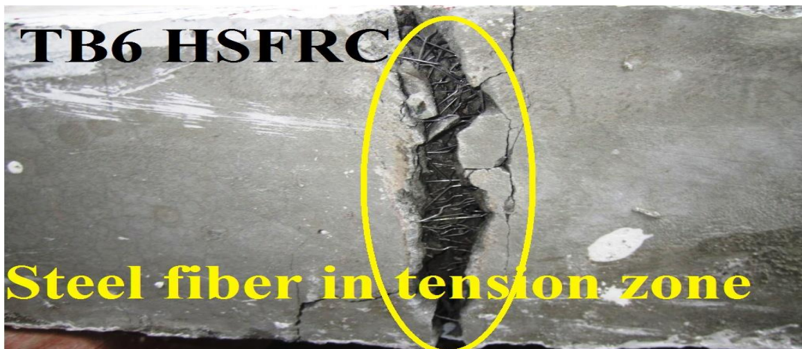
Fig. 4. 23: Failure pattern of 600° C and 900° C heat damaged beams strengthened with HSFRC
