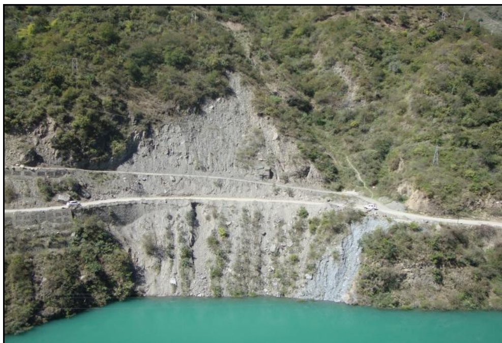
Plate 6.1 View of Debris Slope along the Reservoir
