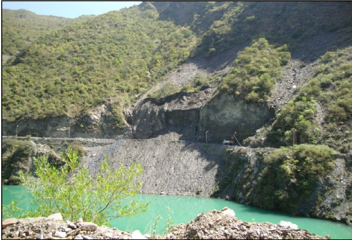
Plate 4.18 View of Slope LBS1 Located 250 m d/s of Zero Bridge
