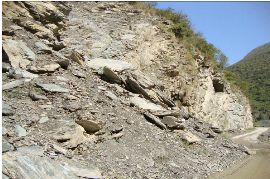
Plate 4.1 A View of Slope RBS1 at 200 m from Zero Bridge
