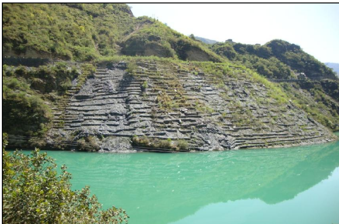
Plate 4.20 A View of Slope LBS3 1.5 km d/s of Zero Bridge (near Chopra Village, Opposite of Pumping Unit)
