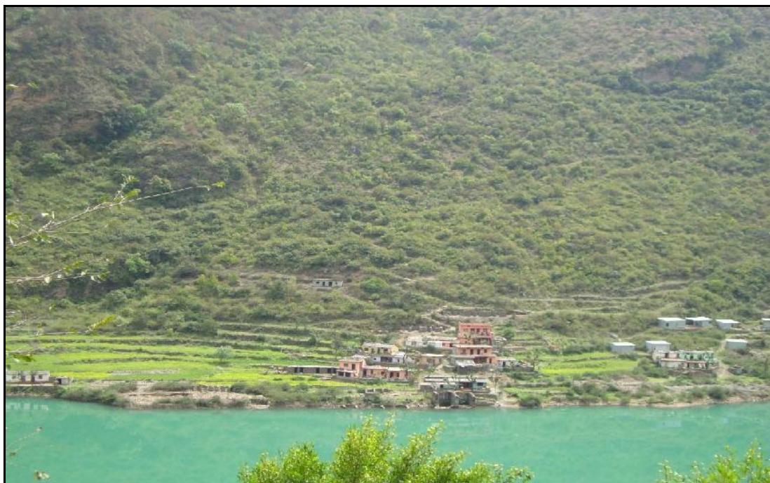
Plate 4.22 A view of Slope LBS5 8.5 km d/s of Zero Bridge (near Bhashon Village just above Old Girder Bridge)
