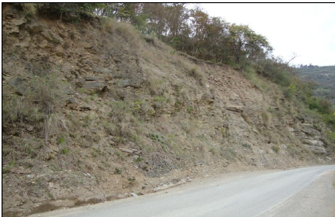
Plate 4.14 A View of Slope RBS14 near THDCIL Guest House
