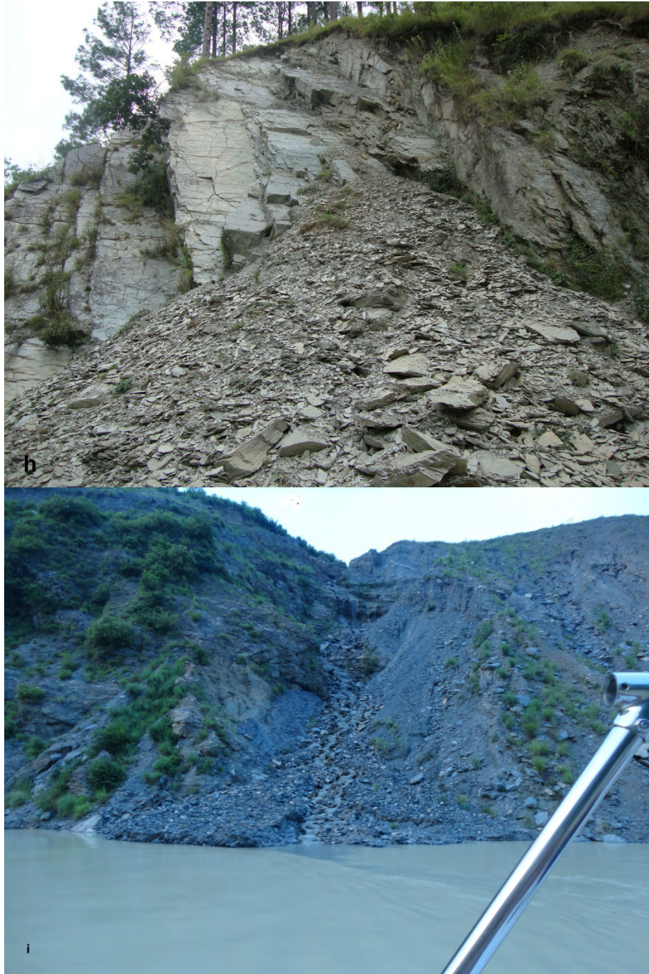
Figure 2.3. Field photographs a) Typical arcuate shape scar of the reservoir induced landslide, b) settlement at risk due to the reservoir induced failures, c) talus slope failure advancing to the upper reaches, d) talus slope failures along the side slopes of the reservoir, e) rotational failure along the road network, f) rotational failure in debris along the road g) a natural slope failure at the ridge, h) slope form of phyllite is subjected to plain failure, i) drainage induced landslide.
