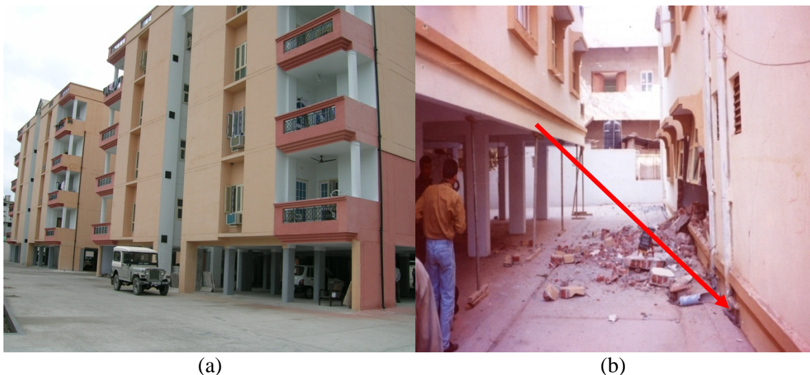
Fig. 1.2 (a) Typical Indian multi-storey buildings with ground storey kept open for parking; (b) failure due to soft/weak storey phenomenon in an open ground storey building during 2001 Bhuj earthquake.
