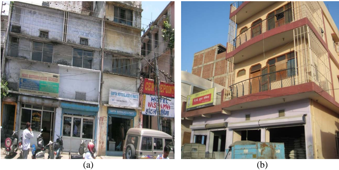
Fig. 1.3 Typical Indian multi-storey residential cum commercial buildings: (a) front kept open for commercial purpose; (b) front kept open and no interior partitions in the ground story, to provide larger spaces for storage.
